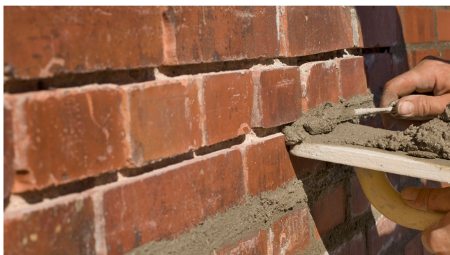
Repointing / The Spruce
